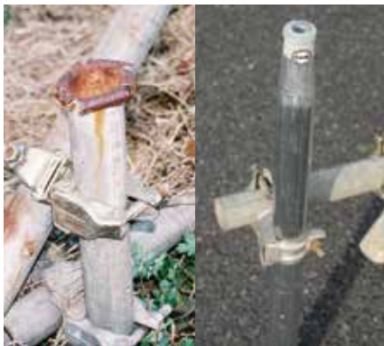
Comparison of construction state between scaffolding pipes and “Kuimaru”
